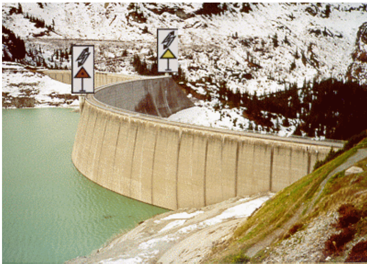
Fig. 6: GOCA GPS-based installation at Kops dam, Austria [4], [5], [6].
