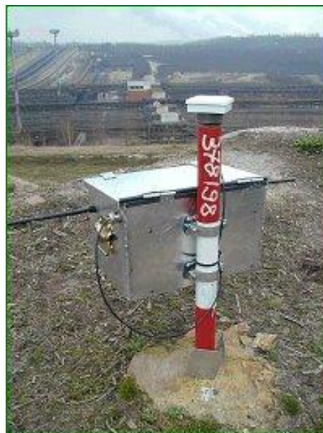
Fig. 1: Example of a GPS receiver and telemetric equipment within a GOCA sensor array in case a slope monitoring in open cast mining at RWE Power AG (see, tab. 1) using the GOCA system
